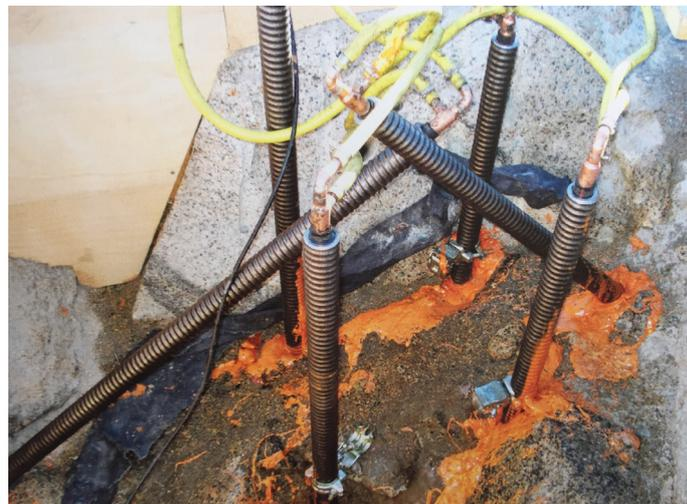
Figure 57. Drilling 6m deep holes in granite to install piles in preparation for steel pillars. Original author
